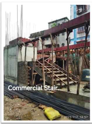
Status: SHUTTERING WORK FOR 1<sup>ST</sup> FLOOR AND COMMERCIAL STAIR IS UNDER CONSTRUCTION.
